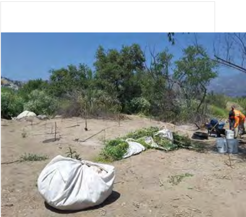
photo_planted stakes and weed removal facing NE.jpg
