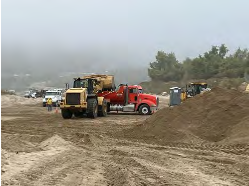
Skiploder_loading_dumptruck_faceS.jpg -118.1715328000001 34.19300415
