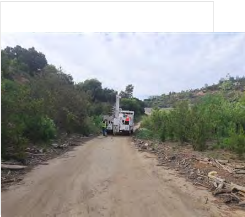
GREGG Drilling conducting hollow-stem auger drilling with tru...
