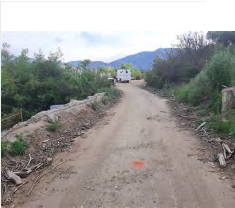
Marked boring location_facingN.jpg
