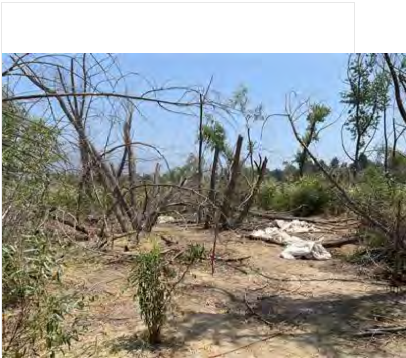
Veg clearing after_mining pit_facing ExNE.jpg
