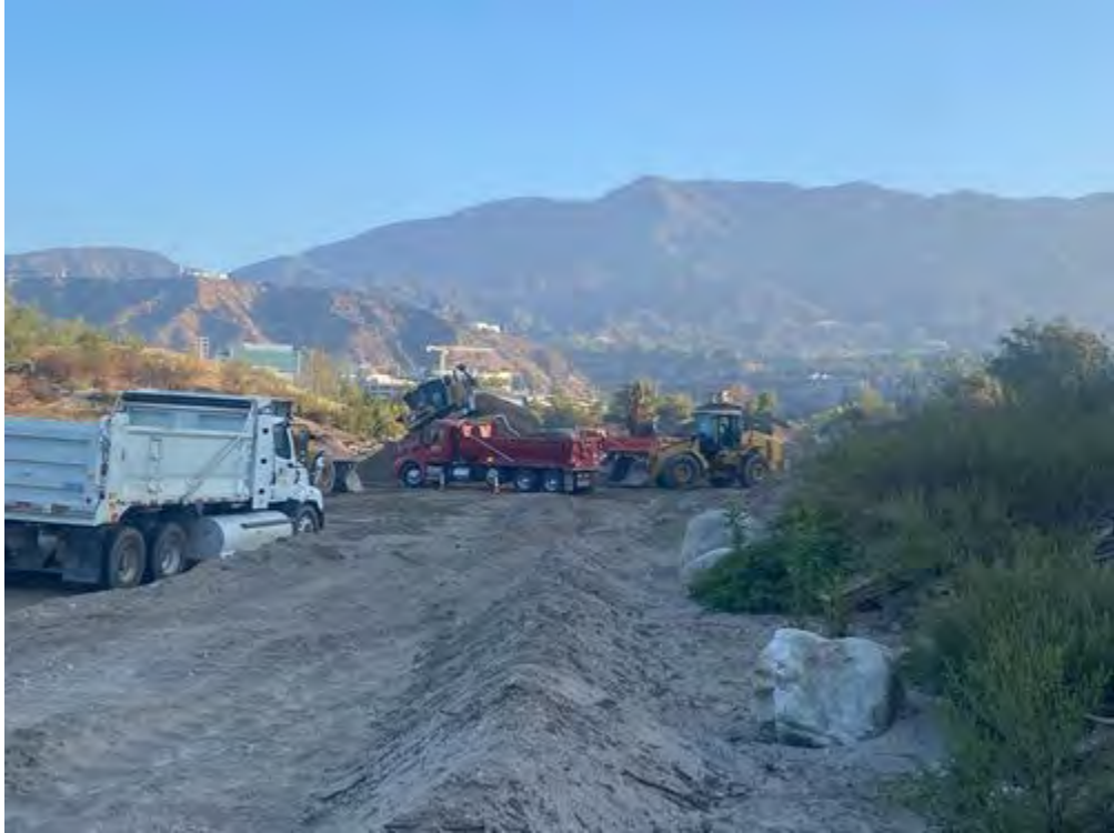
Dozer_loading_sediment_facingNW.jpg -118.17239011111111 34.19188686111111
