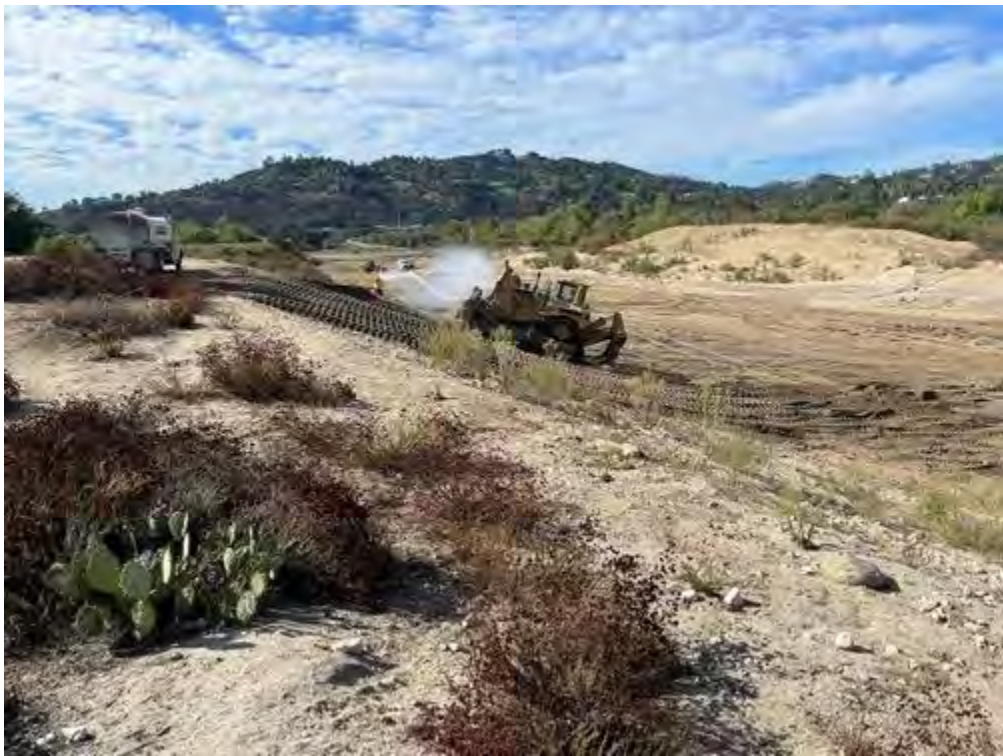
Compacting_north_access_road_facingSW.jpg
