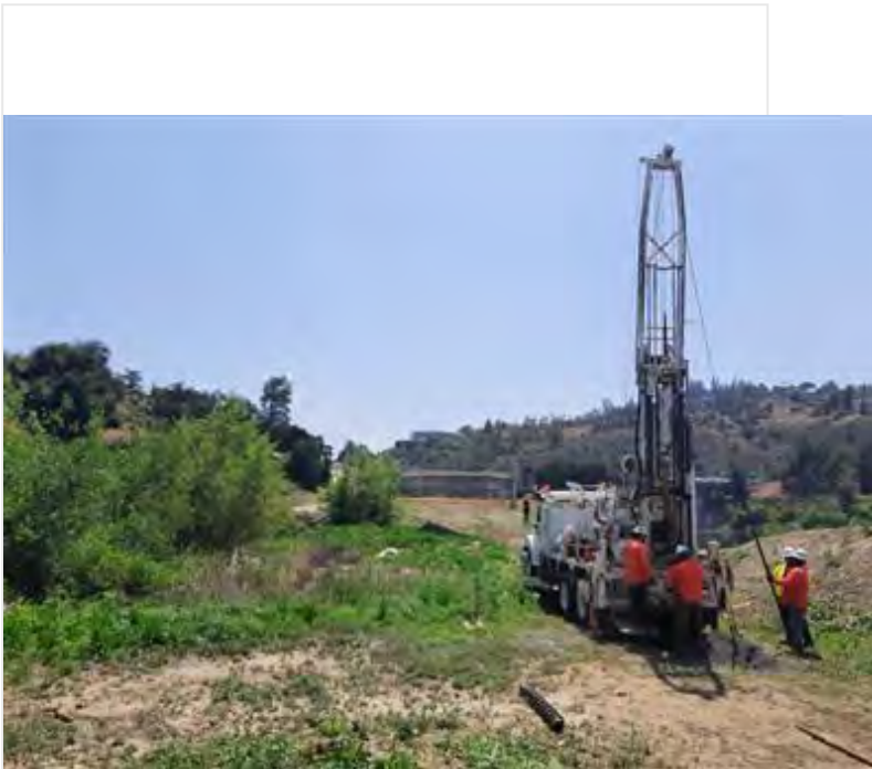
LADWP crew drilling at 2nd boring location near Alta Dena dr...
