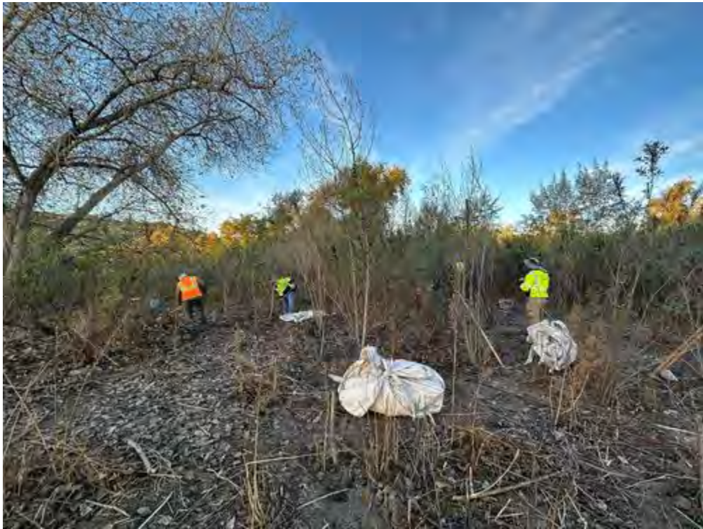
Vegetation Removal facing S during-.jpg
