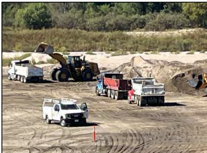
Photo Number: 10 Location: West Side of the Reservoir Description: Dump Trucks Lining up for Sediment Loading
