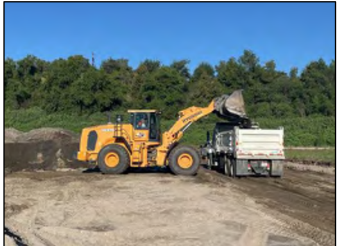
Photo Number: 8 Location: South Side of the Reservoir Description: Front Loader Loading Sediment into Truck
