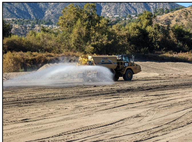
Photo Number: 11 Location: South Side of the Reservoir Description: Water Truck Spraying Reservoir to Prevent Dust
