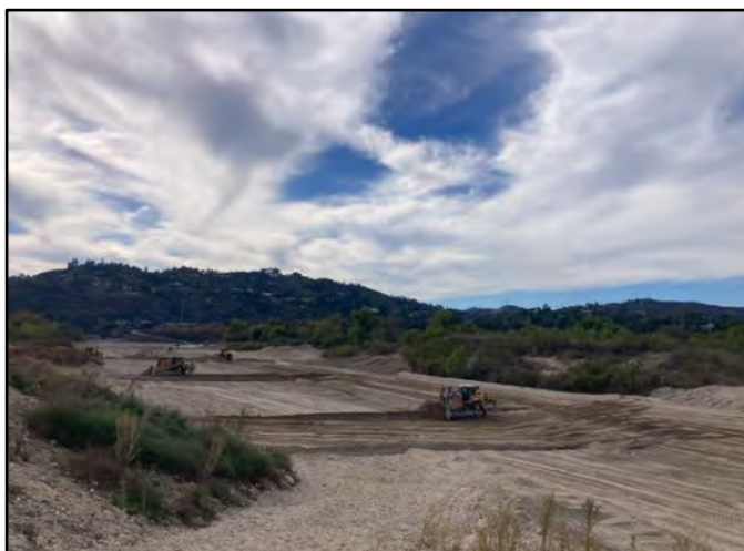
Photo Number: 12 Location: South Side of the Reservoir Description: Grading and Shaping East Slopes
