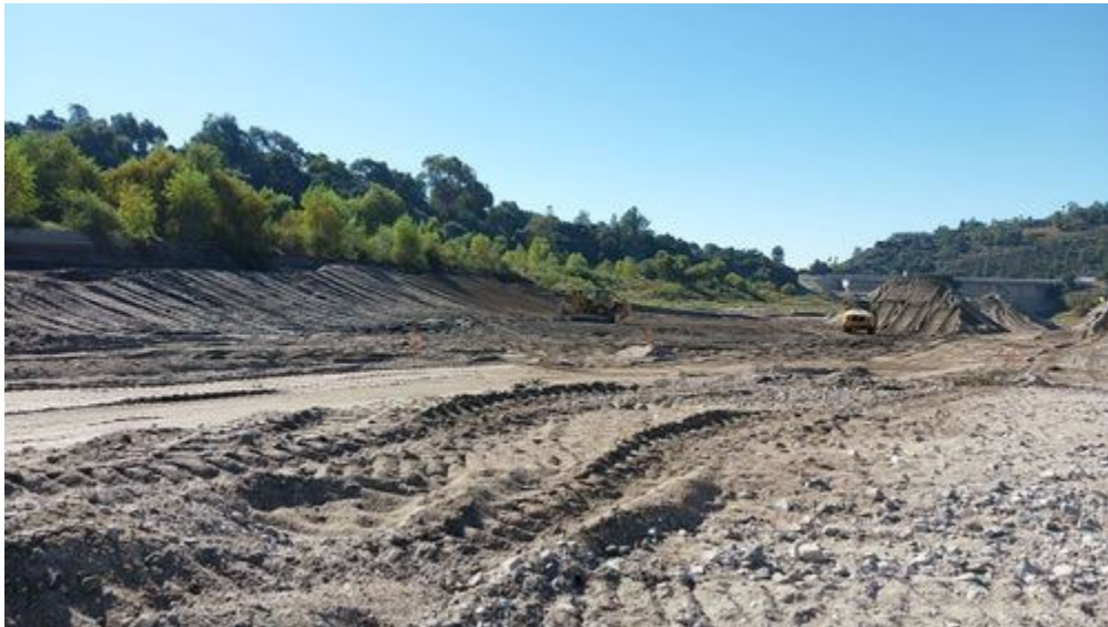
bulldozer_compacting_bank_reconstruction_facingSouthSoutheast.jpg
