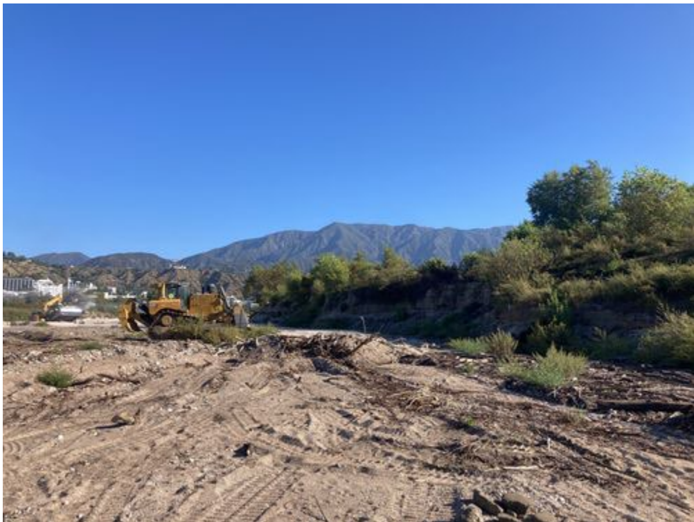
Beginning_of_grading_for_cliff_stabilization_facingNortheast.jpg -118.1729711388889 34.1896280916666
