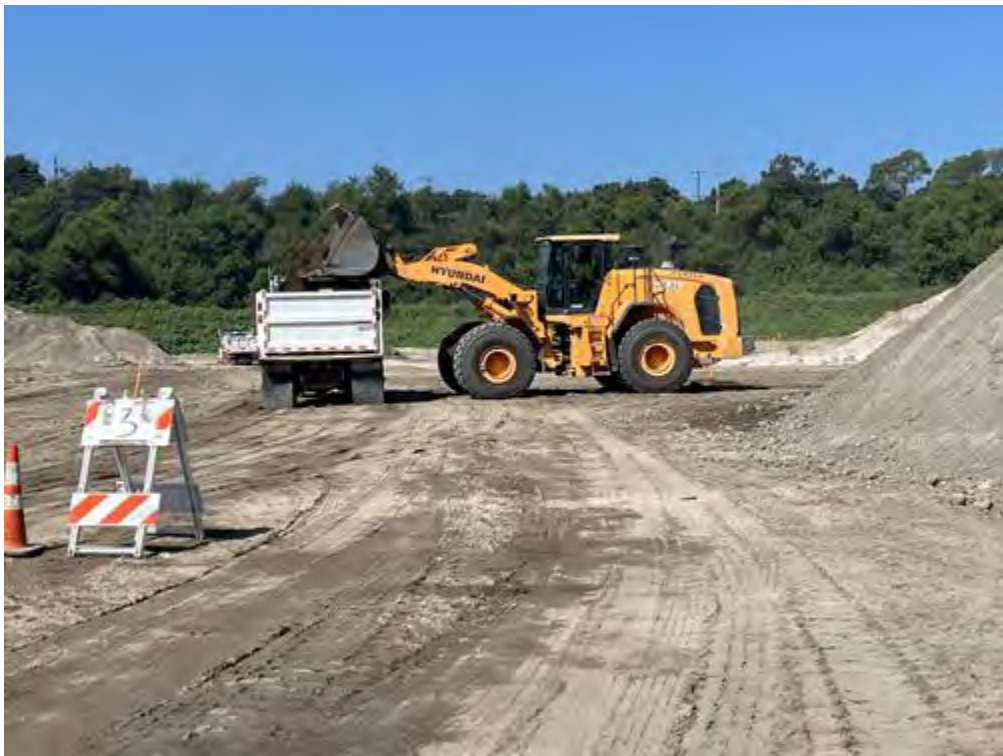
Skiploder_loading_soil_on_dumptruck_faceWest.jpg -118.17420268055557 34.18813755555555
