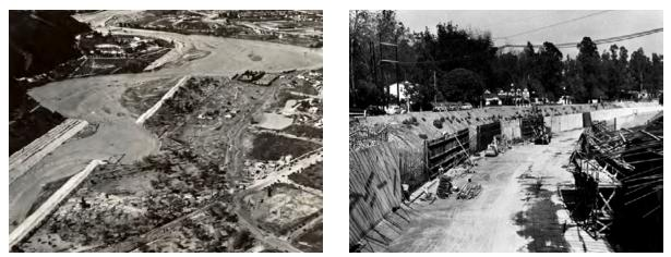
Figure 50. (Left) This aerial view of the 1938 flood from above Victory Blvd shows breaches in paved levees in and below a sharp curve in channel alignment. Source: USACE, 1938.
