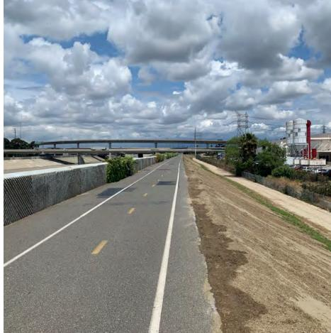
Figure 62. The lower river's parapet walls, such as these shown at river mile 10.1, were installed in the late 1990s in order to increase the channel capacity to greater than the 1% event. Source: OLIN, 2019.
