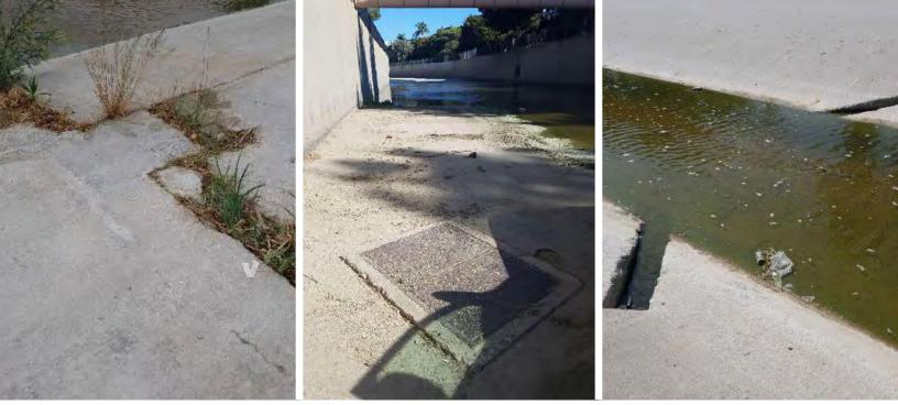
Figure 367. Channel lining, sub-drain hatch, and weep holes along the side of the LA River channel. Source: Geosyntec, 2018.
