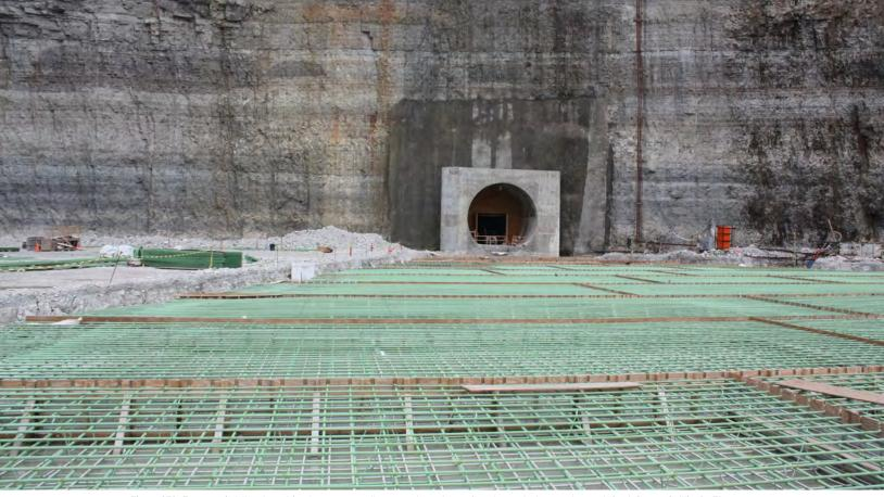
Figure 279. Excess rainfall and combined sewage overflow runs through a series of tunnels deep underneath Cook County in Illinois. The water discharges into large reservoirs where it is held until it can be treated and released back into the water system. Source: OLIN, 2019.
