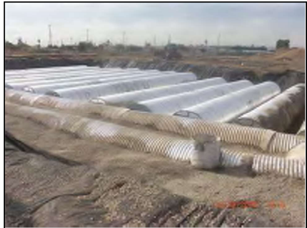
Underground Infiltration Units Lowe's, Pacoima
