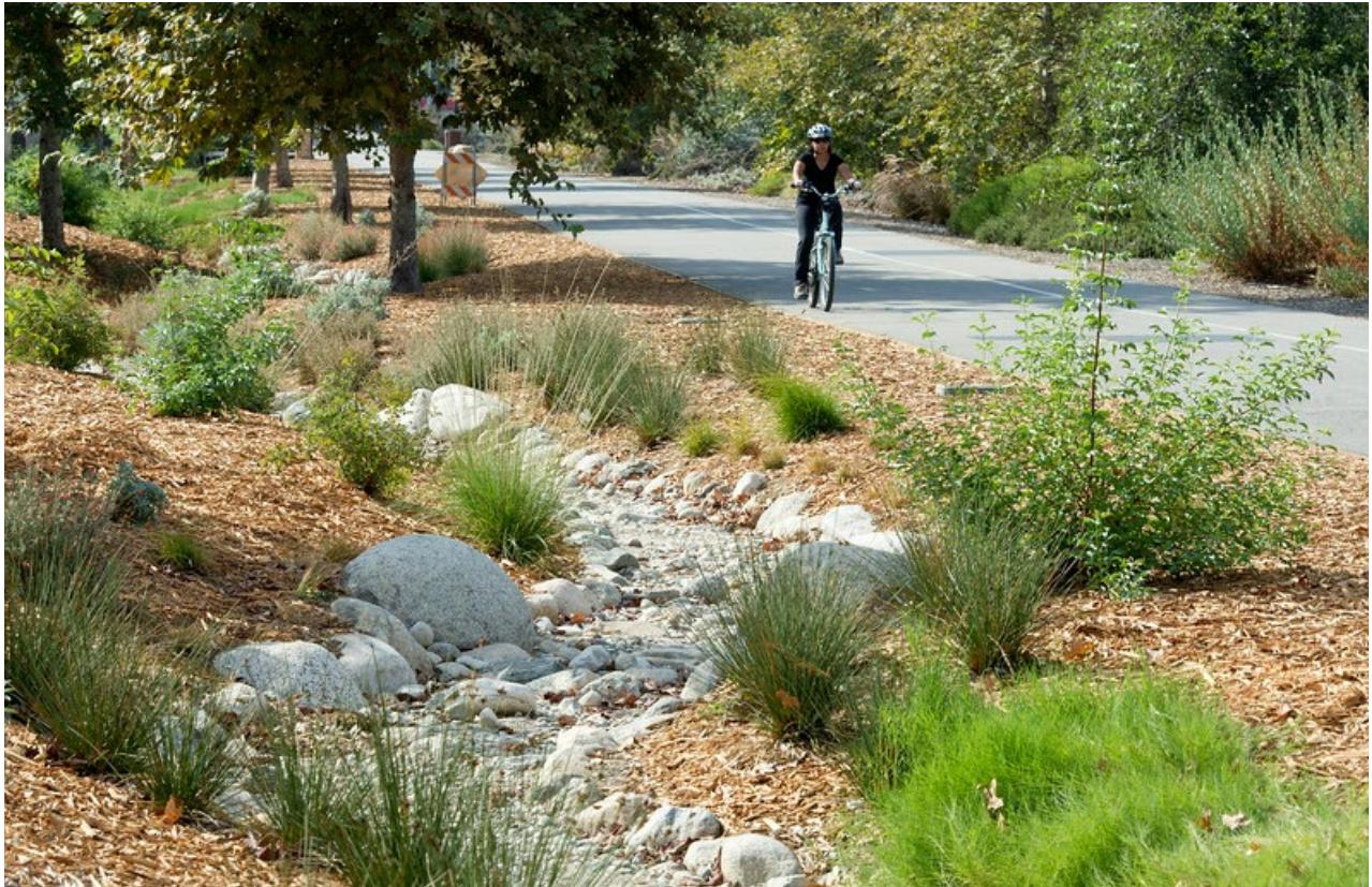
Figure 11-1. Example bioretention swale next to greenway
