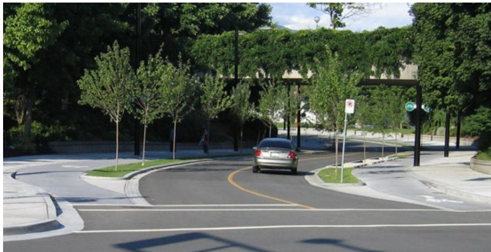
Figure 7-4. Example Class IV grade-separated bikeway in Vancouver, British Columbia
