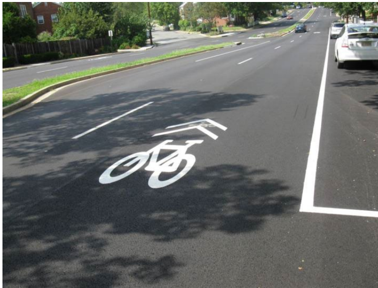
Figure 6-1. Example Class III bikeway installed in Arlington, Va.
