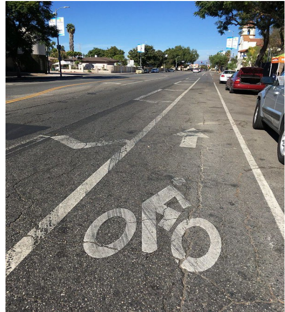
Figure 5-1. Class II bikeway includes dedicated ROW for bicyclists designated with a striped line and/or painted buffer zone
