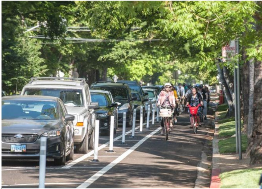
Figure 7-1. Example Class IV bikeway with flexible posts and adjacent parking
