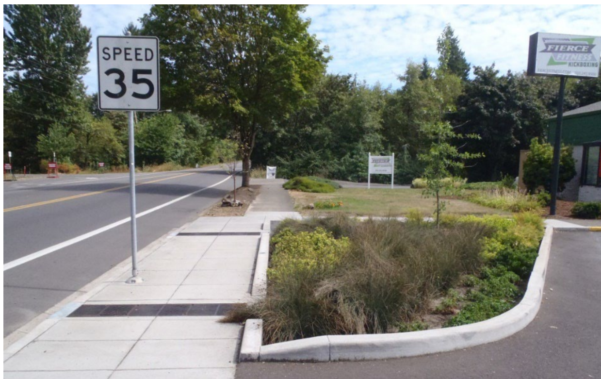
Figure 11-3. Example stormwater planter with surface inflow
