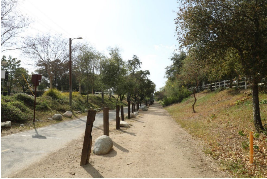
Figure 10-10. Minimal wooden post and boulder barrier between equestrian trail and bikeway path in Duarte
