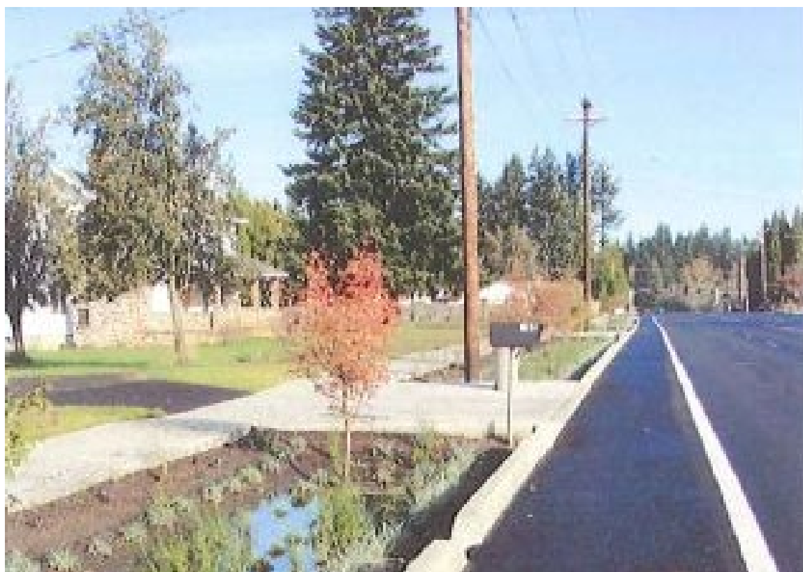
Figure 11-9. Permeable asphalt bike lane and roadside bioswale
