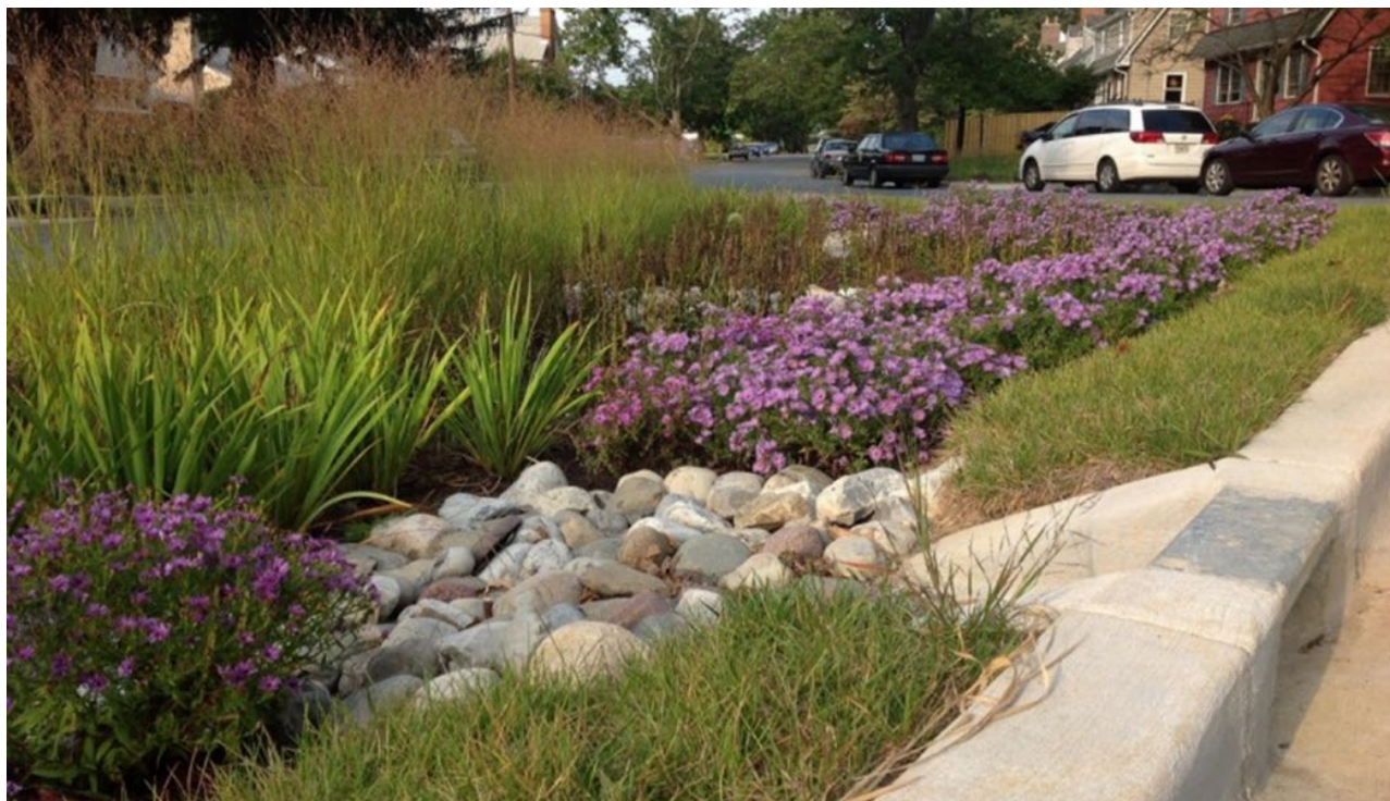
Figure 11-2. Example bioretention basin with surface inflow
