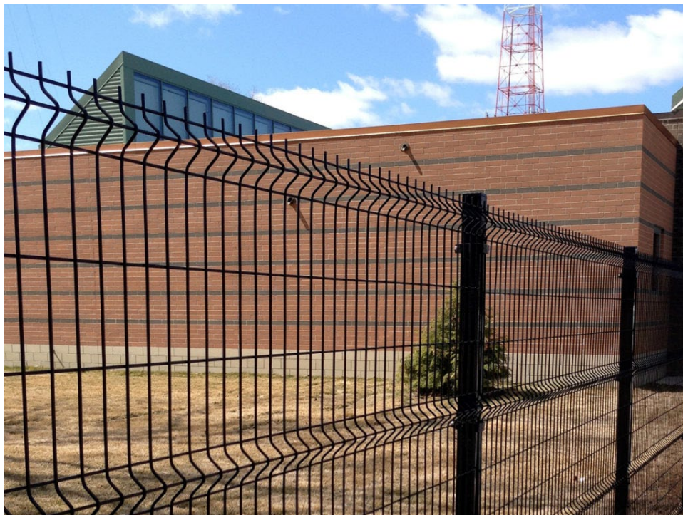
Figure 10-3. Standard welded wire (Omega Style) fence located between the residential property and the proposed greenway
