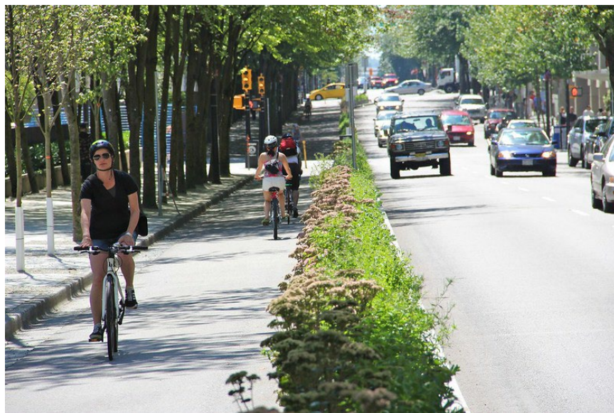
Figure 7-6. Example of an inflexible barrier (street planter) for a Class IV bikeway
