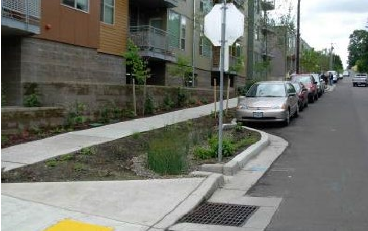
Figure 11-4. Example curb extension with surface inflow
