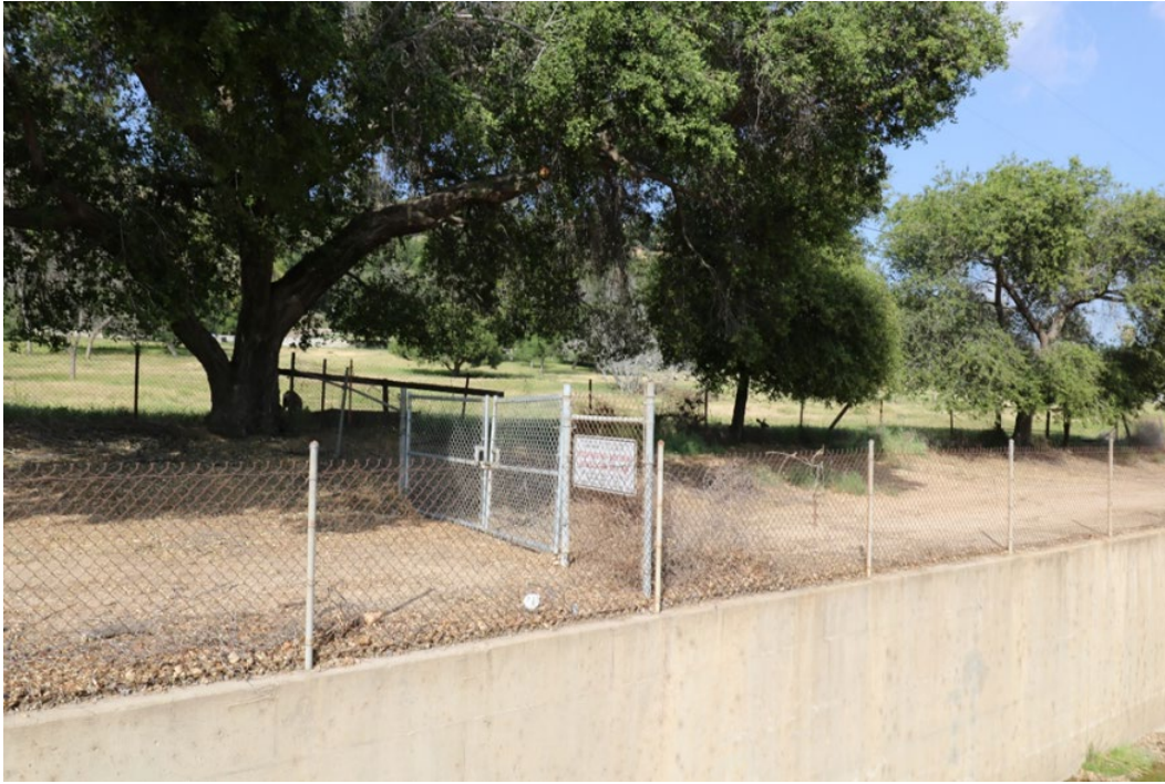
Figure 10-21. Existing double fence gate in Duarte
