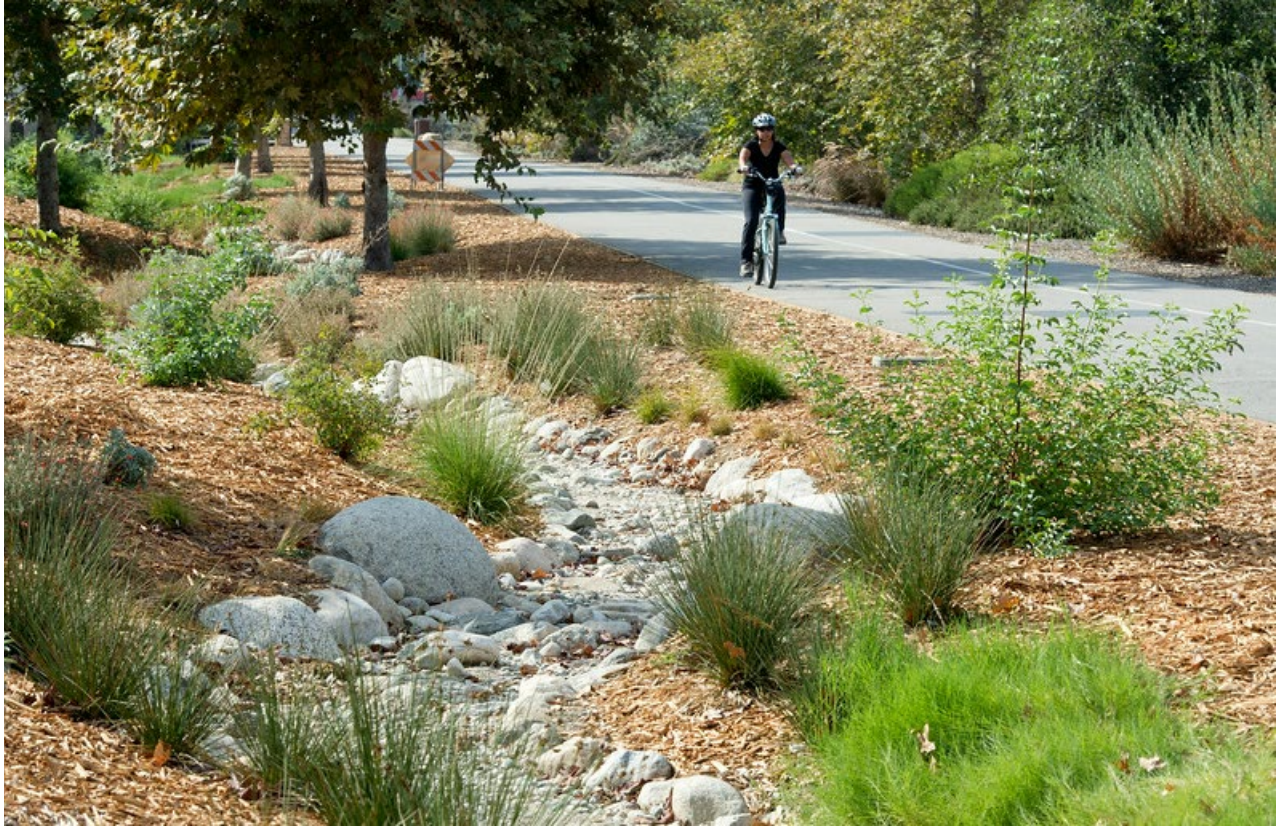
Figure 11-1. Example bioretention swale next to greenway
