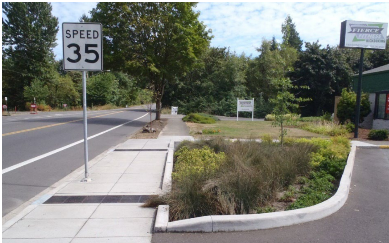
Figure 11-3. Example stormwater planter with surface inflow
