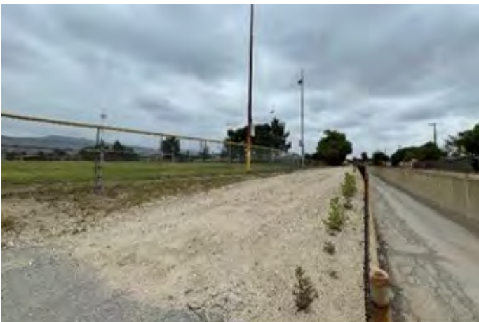
Figure 1-5. Example District channel ROW suitable for conversion to a bike path or multi-use path. This site is situated between the San Dimas Wash and an existing park, Hollenbeck Park, where opportunities for offsite stormwater management have been identified.
