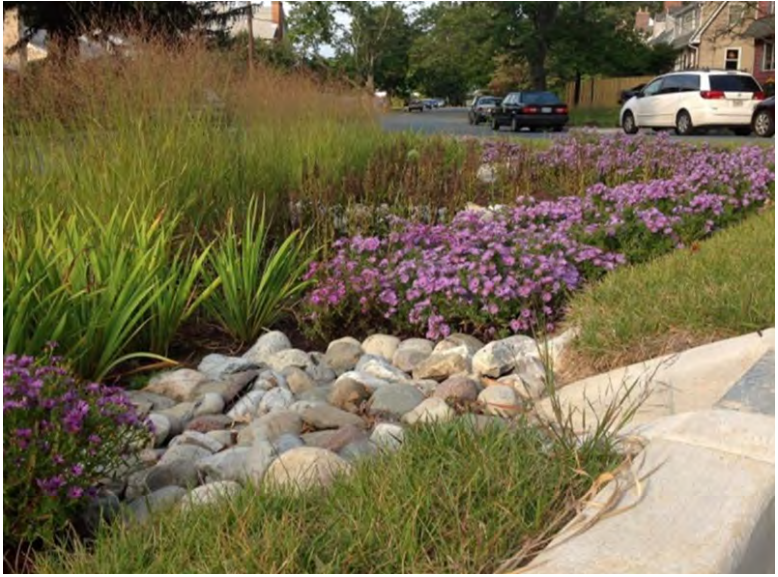
Fig 1-24. Example bioretention basin with surface inflow
