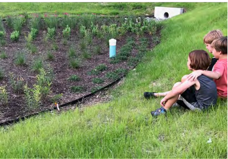
Fig 1-22. Example bioretention basin with pipe inflow
