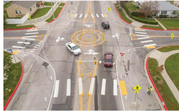
**Temporary Roadway Enhancements** such as paint and flexible posts/bollards are typically less expensive than concrete and may be installed to enhance traffic safety.
