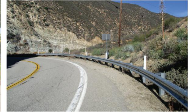
**Guardrail** is installed to reduce the severity of run-off road collisions. However, guardrail can reduce crash severity only for those conditions where striking the guardrail is less severe than going down an embankment or striking a fixed object.
