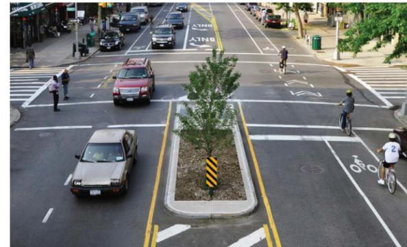
**Roadway Reconfigurations** typically reduce the number of vehicular travel lanes and may reallocate space to pedestrians and bicyclists and allow room for vehicle turning lanes. Narrower traffic lanes may also contribute to slower speeds while the addition of roadway trees along corridors can have a traffic calming effect.
