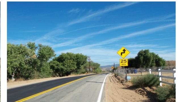
**Curve Warning Signs** provide emphasis and guidance for a change in horizontal alignment. Advisory speed signs may be used to supplement warning signs.
