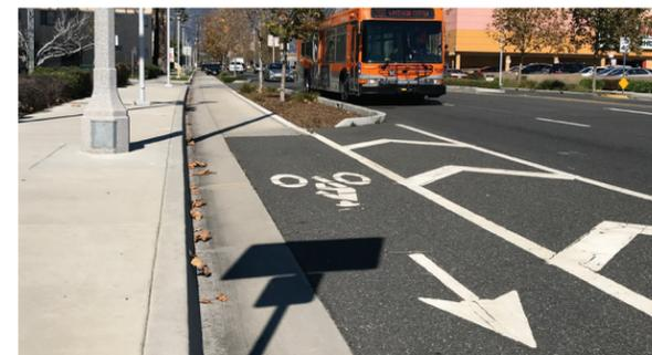
**Separated Bikeways** provide physical separation between bicyclists and traveling motorists.
