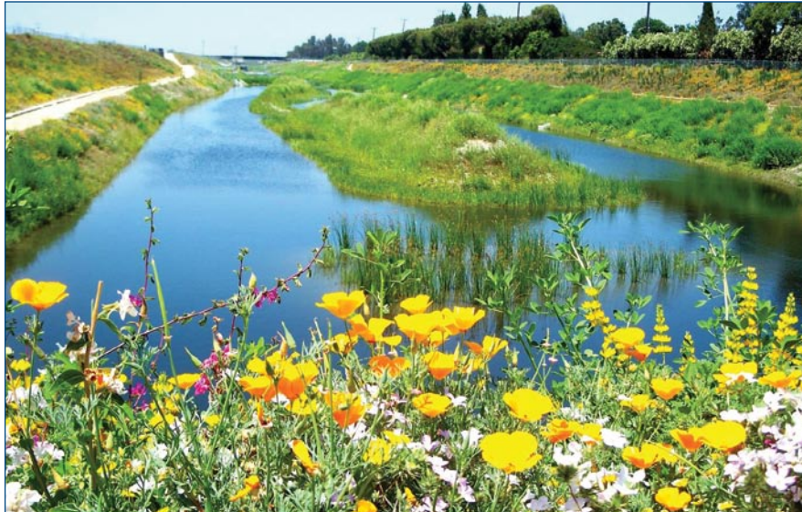
The east basin of the Dominguez Gap Wetlands naturally treats from 2-3 cubic feet per second (1.3 to 3.2 million gallons a day) of stormwater and urban runoff—enough water to fill five Olympic-size swimming pools.
