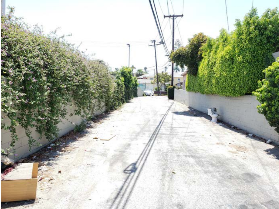
Photo 5—View to the southwest from the View Park Green Alley Site’s eastern Site boundary.
