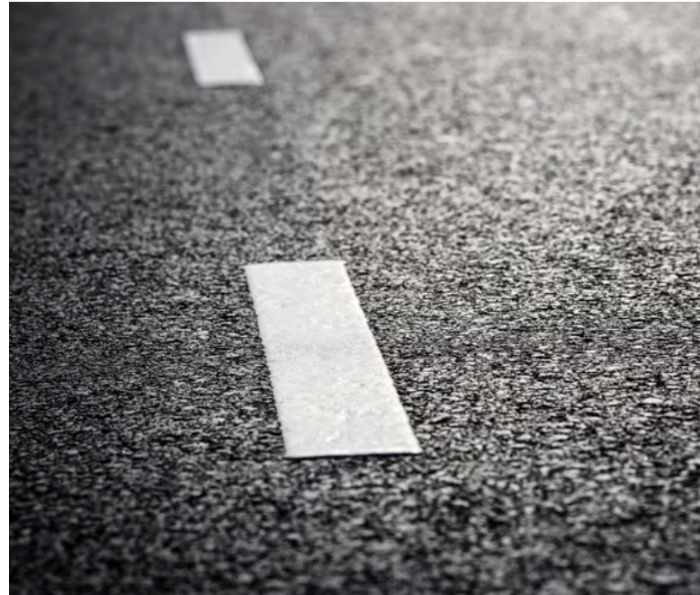
Figure 119. Thermoplastic paint is a durable option for pavement markings on asphalt. Source: LeManna, Shutterstock.com, 2020.
