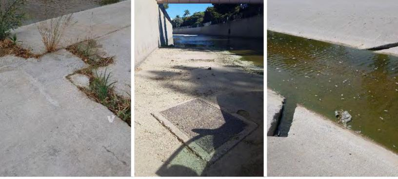
Figure 352. Channel lining, sub-drain hatch, and weep holes along the side of the LA River channel. Source: Geosyntec, 2018.
