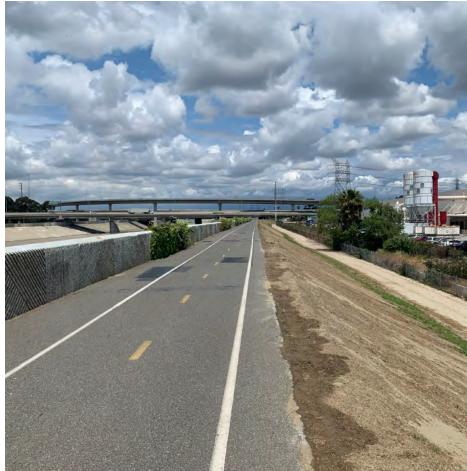
Figure 57. The lower river's parapet walls, such as these shown at river mile 10.1, were installed in the late 1990's in order to increase the channel capacity to greater than the 1% event. Source: OLIN, 2019.
