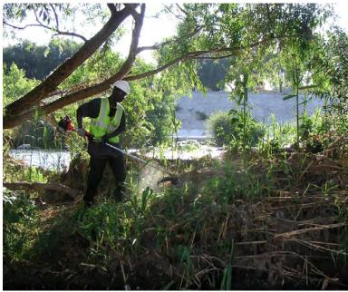
Figure 143. A worker removes invasive plant material from the channel near the Glendale Narrows, a maintenance practice that helps to increase the flood capacity of the LA River. Source: US Army Corps of Engineers, LA River Arundo Removal, 2004.
