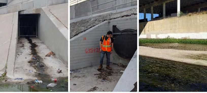
Figure 353. Outfall, soft bottom sediment and vegetation build-up inspection, and concrete bottom build-up. Source: Geosyntec, 2018.
