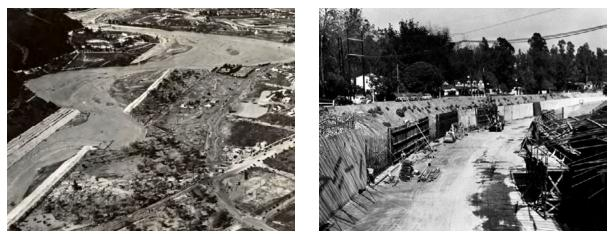
Figure 45. (Left) This aerial view of the 1938 flood from above Victory Blvd, shows breaches in paved levees in and below a sharp curve in channel alignment. Source: USACE, 1938.
