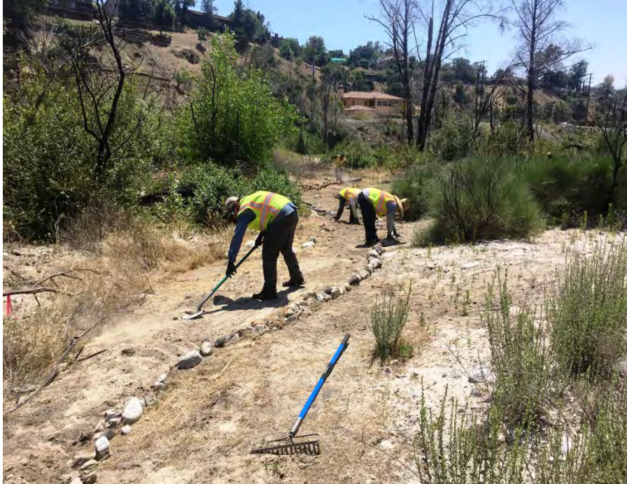
Photo 3: Crew members cutting, grading, and using stones to delineate the eastern trail section, on June 7.
