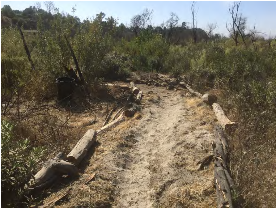
Photo 6: Section of the eastern trail realignment after widening. The trail now allows easier passage of equestrian riders traveling in opposite directions, reducing the need to ride off trail.
