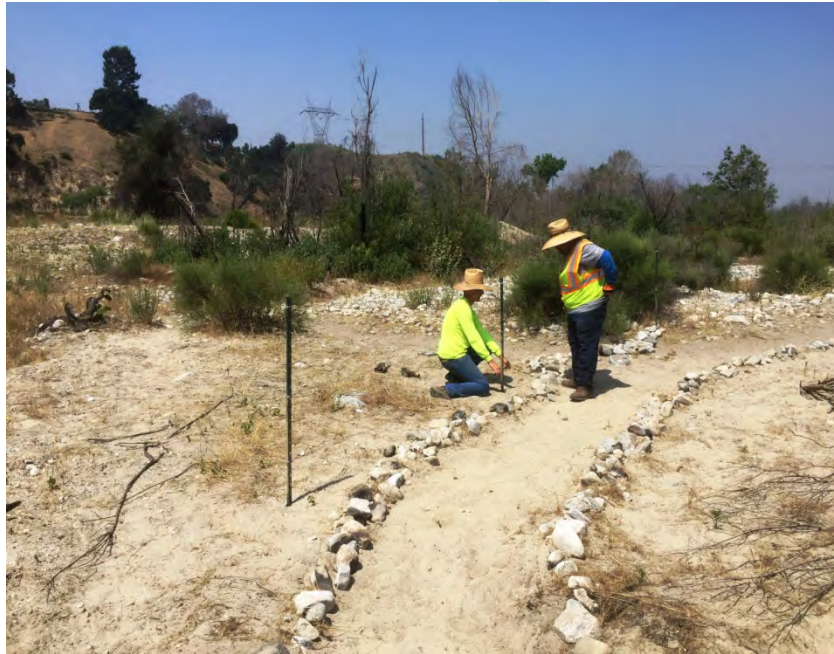
Photo 7: Crew members installing T-posts and three-wire fencing at the western creek crossing trail closure, on July 13.
