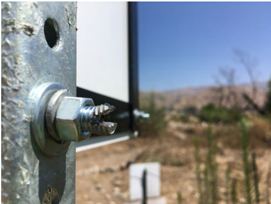
Photo 22: Example of how sign bolts were split and flared to discourage theft.
