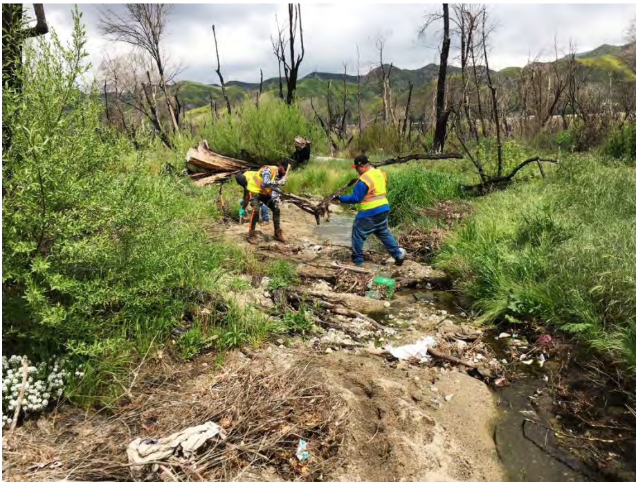
Photo 4: Continuation of snag root removal, clearing debris and garbage, and grading on April 4.
