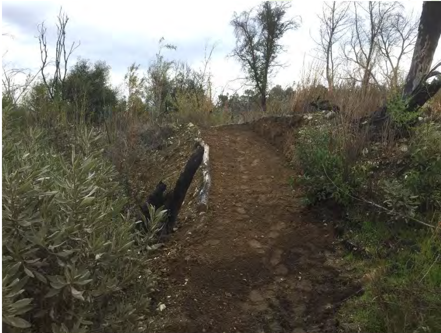
Photo 7: Ramp after trail widening. The wider trail will provide more room for equestrian riders to pass one another and reduce the need to ride off-trail.
