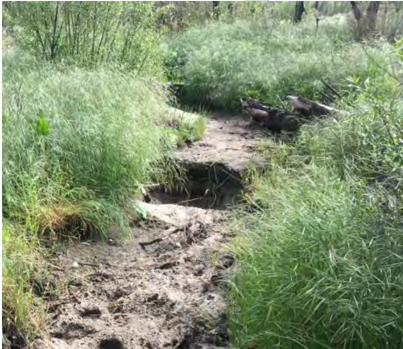
Photo 4: Before backfilling and grading a swale depression.
