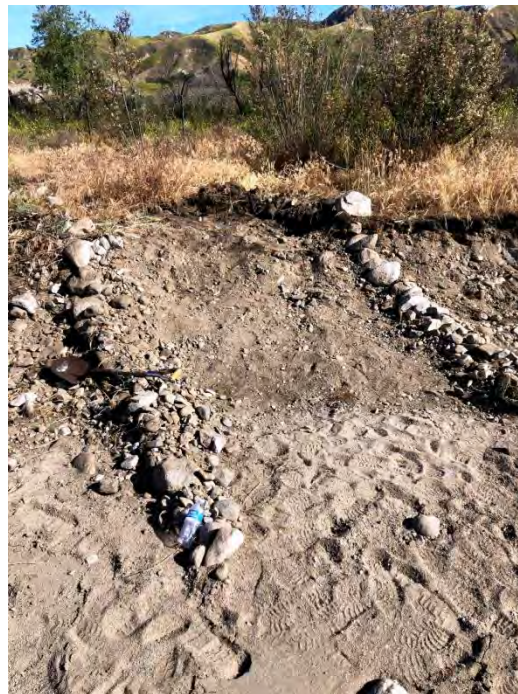
Photo 6: After completing the grade for the new crossing point, crew members used the exposed rocks to delineate the continuation of the trail, on April 18.
