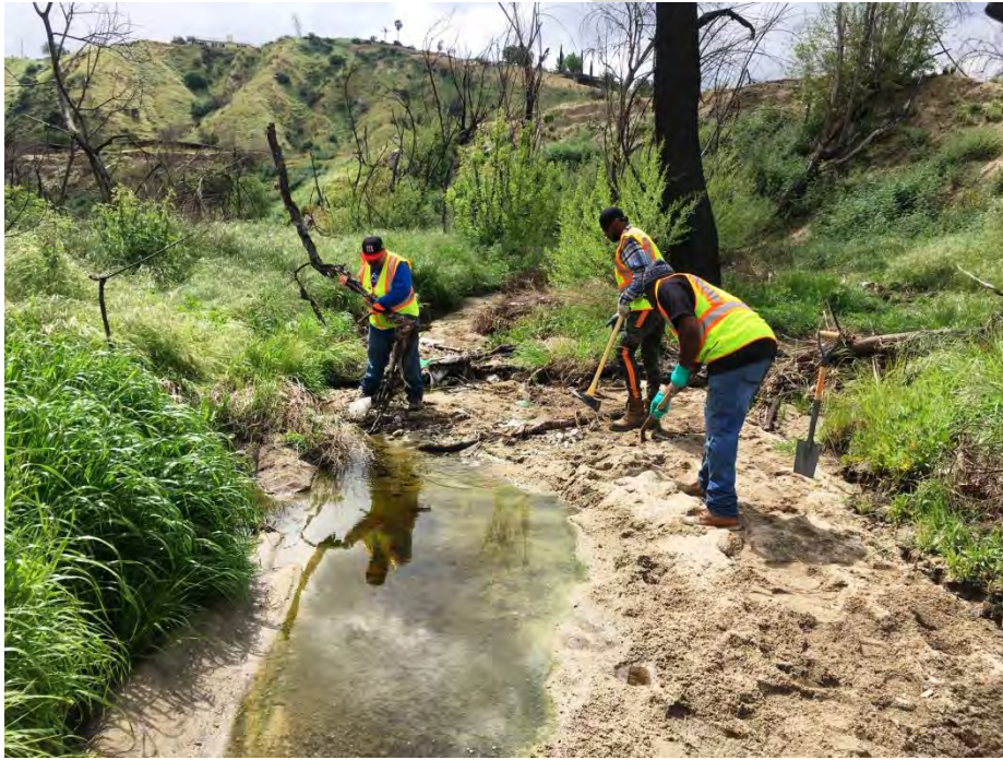
Photo 3: On April 4, crew members removed exposed snag roots, cleared the area of garbage, and graded the area to safely pass around a seep.
