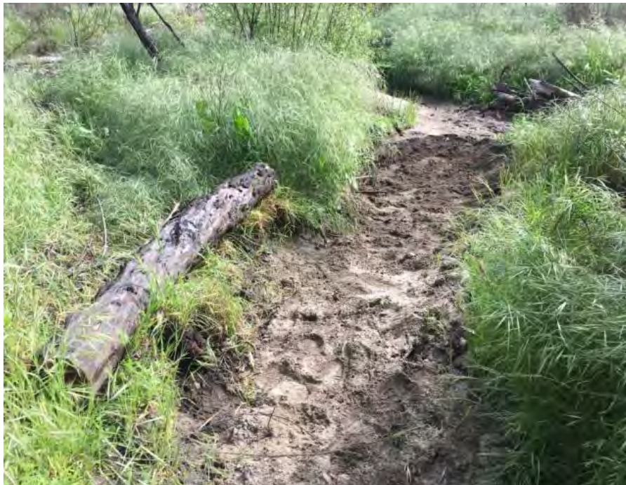
Photo 4: After backfilling and grading a swale depression. Felled debris was used to delineate the authorized trail.
