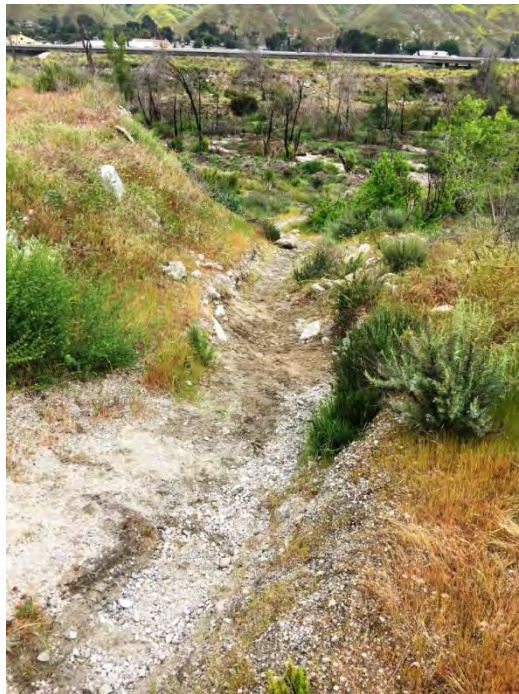
Photo 2: After the trail was cleared of boulders, backfilled, and graded, on April 4.
