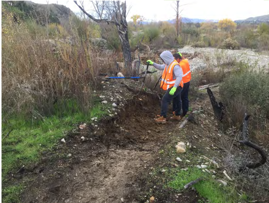
Photo 5: Crew members digging out the slope to widen a ramp within the eastern trail realignment.
