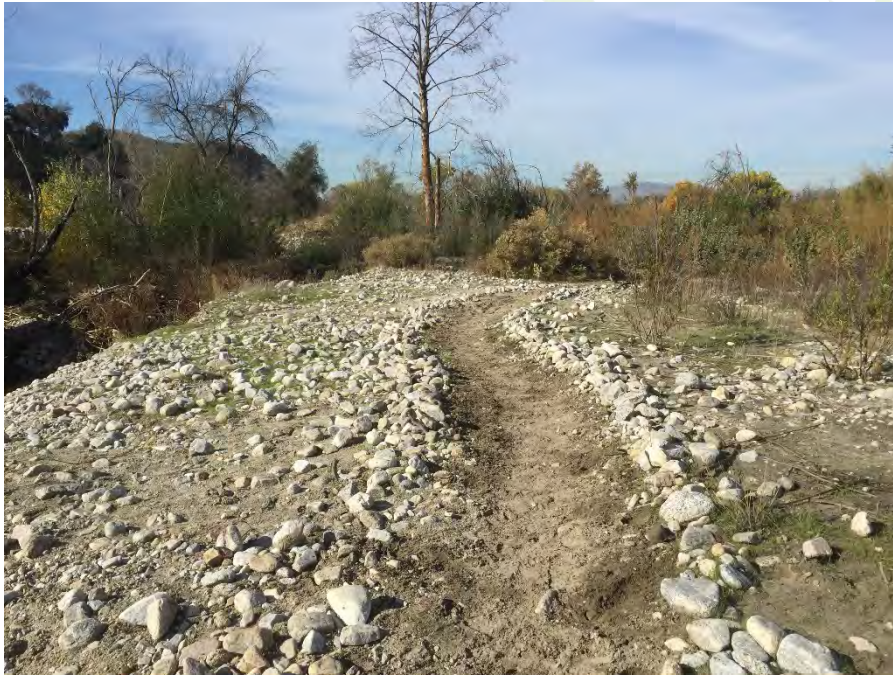
Photo 9: Rocks were removed and used to clearly delineate authorized trails to minimize off-trail riding, and provide for safe equestrian travel.
