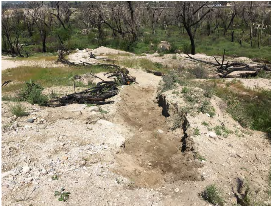
Photo 6: The equestrian entry point affected by washout, after being backfilled and graded. Felled debris in the surrounding area was used to delineate the authorized trail entry and course.
