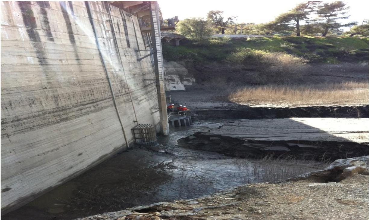
A-4 Sediment Threatening Sluice Gate Post-Station Fire
