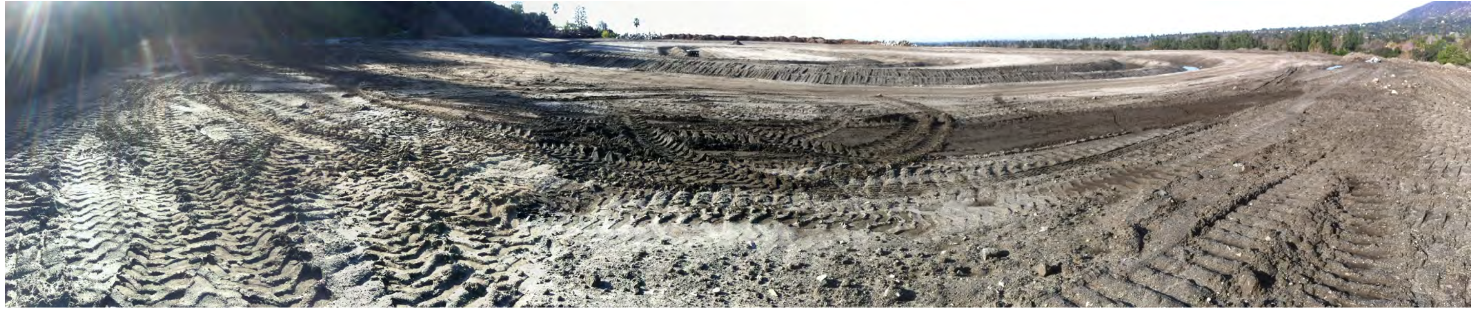
January 2013. Photo Station No. 4.
