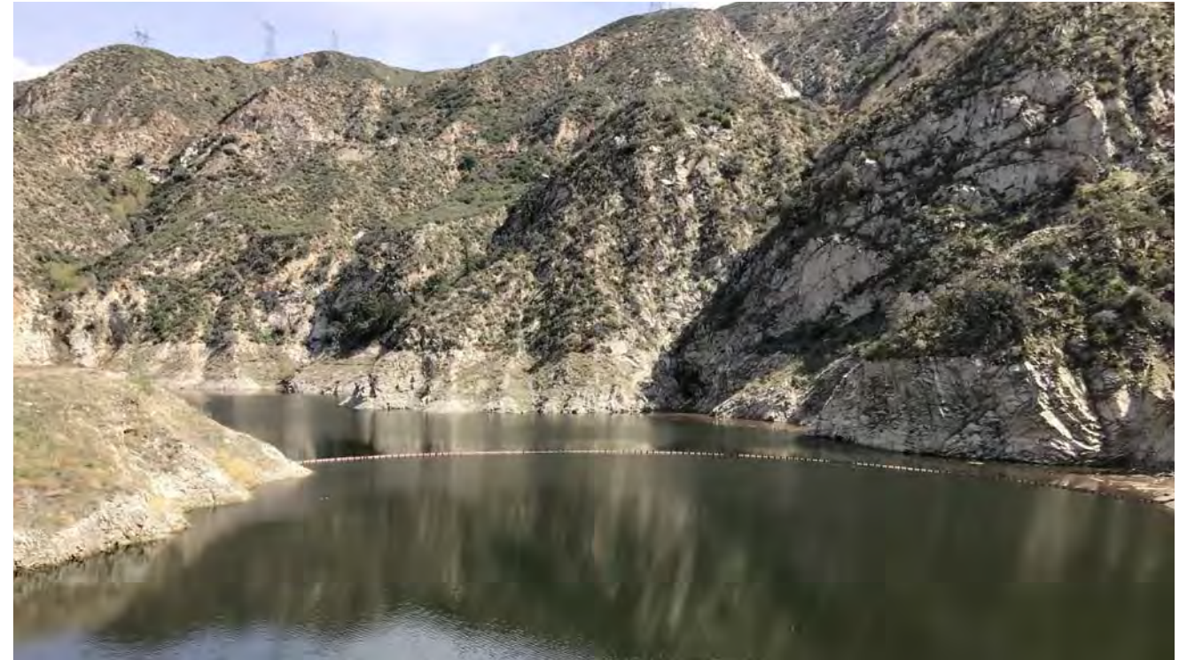
Photo 2: Photo depicts water within BTR behind dam structure looking east.
