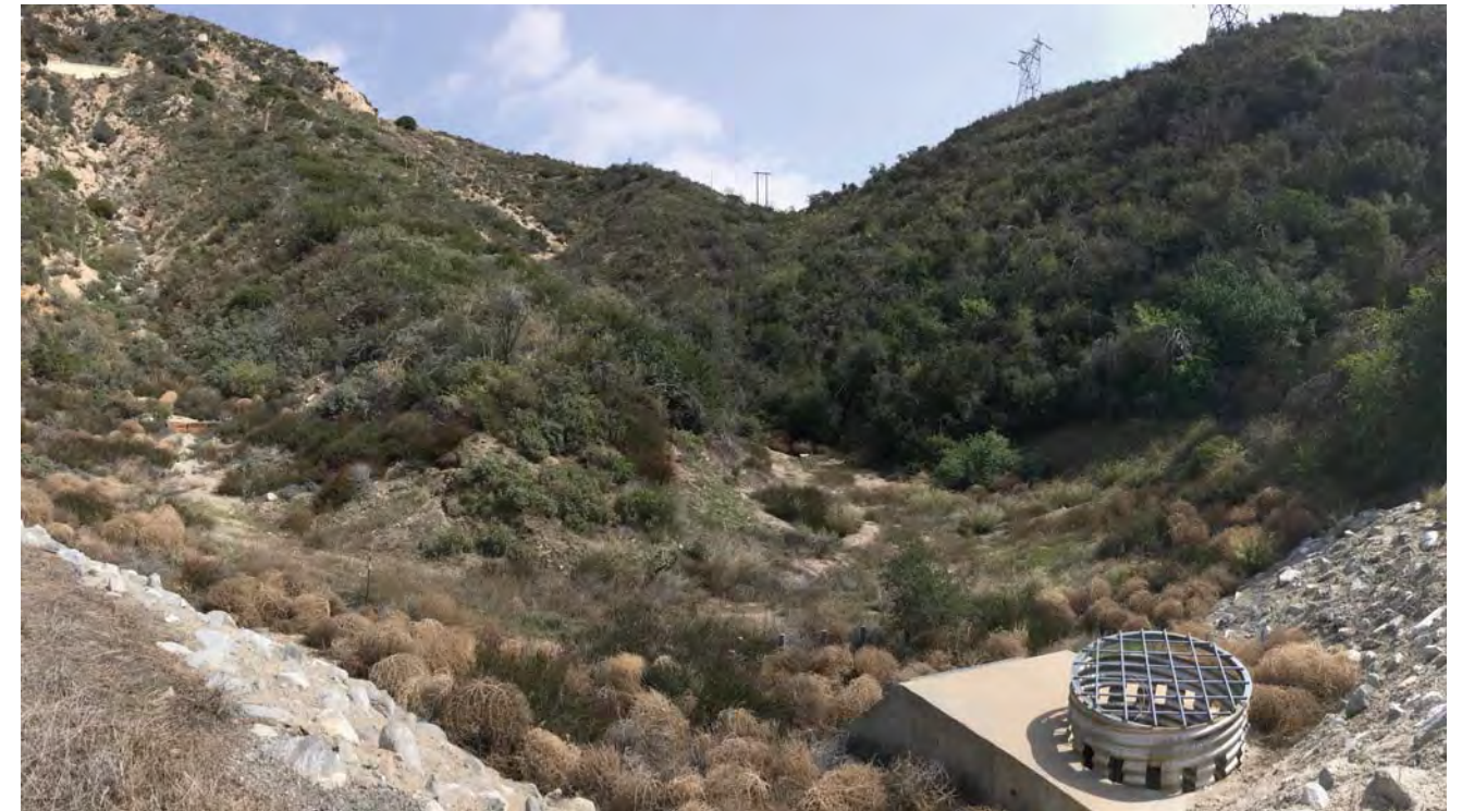
Photo 8: Photo depicts remaining capacity in far eastern edge of Maple Canyon SPS, looking east.
