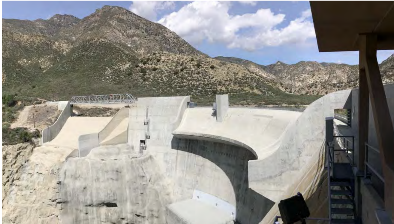
Photo 1: Photo depicts BTR dam structure looking north.
