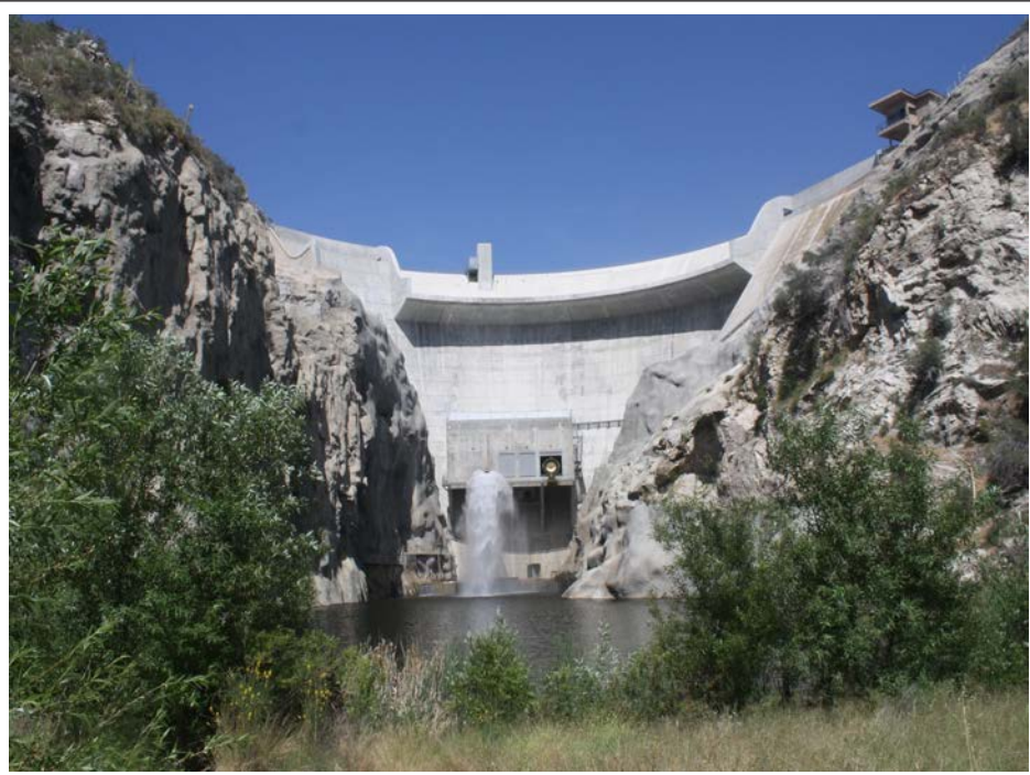
Photo 16 - Photo of Big Tujunga Dam and plunge pool from the Dam Access Road, looking upstream. Photo shows the developed Dam, cliffs on each side of the Dam, open water of the plunge pool, and white alder grove-willow thicket in the foreground.
