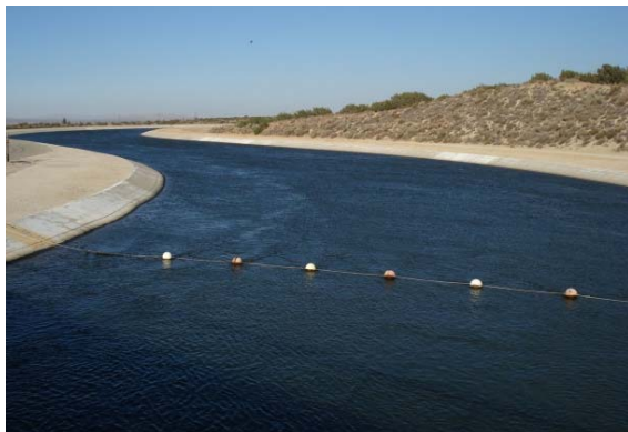
The State Water Project delivers imported water to the Antelope Valley.
