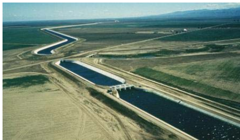
THE CALIFORNIA AQUEDUCT
