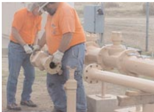
Field staff install an ASR injection line.
